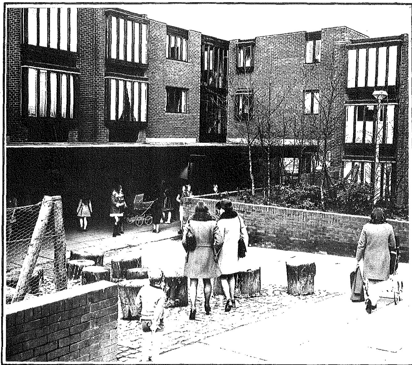
Plate 14. The hub of Halton Brook — pensioners flats above the shopping centre
